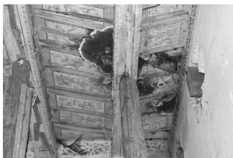
Fig. 4. Biological corrosion of ceilings: a) corrosion caused by a lack of the appropriate atmospheric conditions, b) corrosion caused by the direct impact of water
