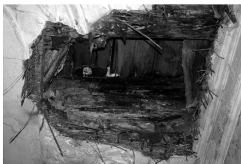
Fig. 4. Biological corrosion of ceilings: a) corrosion caused by a lack of the appropriate atmospheric conditions, b) corrosion caused by the direct impact of water
