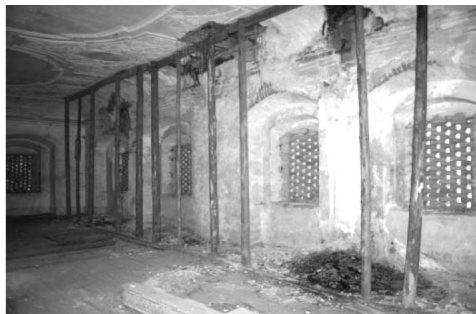
Fig. 3. Damage to ceilings of successive floors caused by the local impact of water: a) damage on the II floor, b) damage on the I floor
