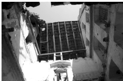
Fig. 5. Ceiling damage: a) absence of ceilings that collapsed along with the roofing, b) fire damage
