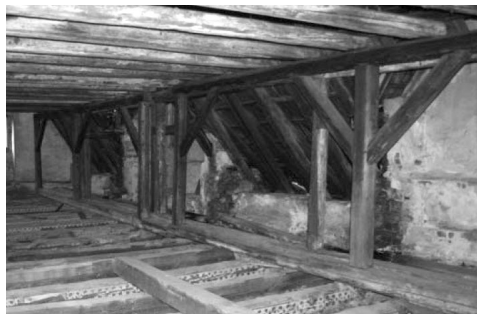
Fig. 3. Damage to ceilings of successive floors caused by the local impact of water: a) damage on the II floor, b) damage on the I floor
