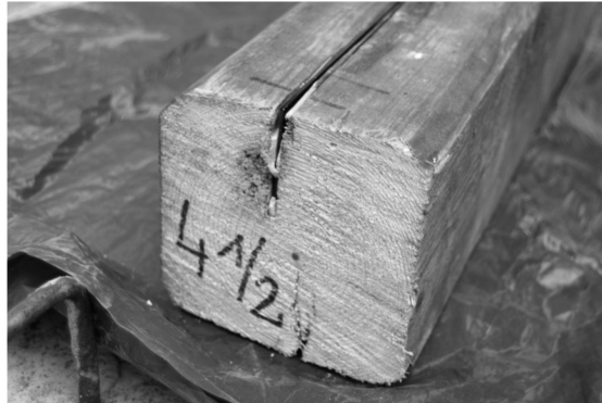
Fig. 13. Reinforcement of ceiling beams in the palace in Gorzanów
