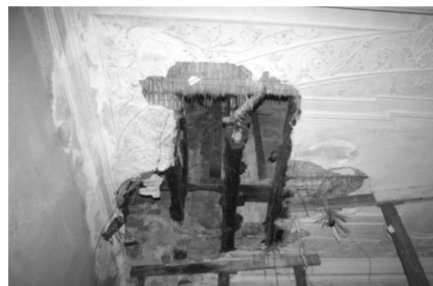
Fig. 5. Ceiling damage: a) absence of ceilings that collapsed along with the roofing, b) fire damage
