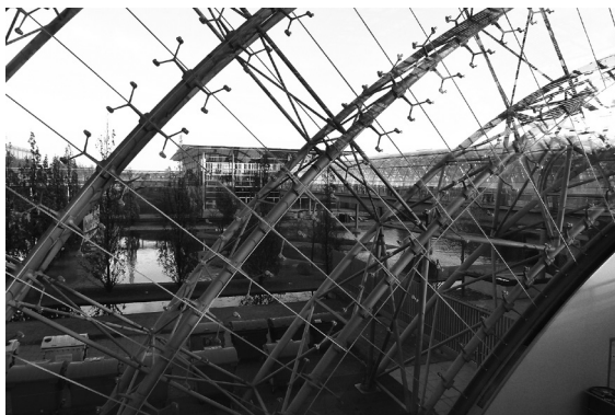
III. 15. Leipzig, the Glass Hall – a fragment of the construction of the gable end (photo by the author)
