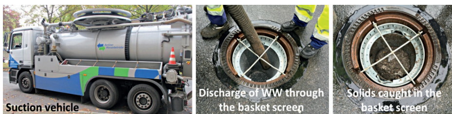
Fig. 6. From left to right: Suction vehicle, wastewater being discharged into the basket screen, basket screen retaining the solid
