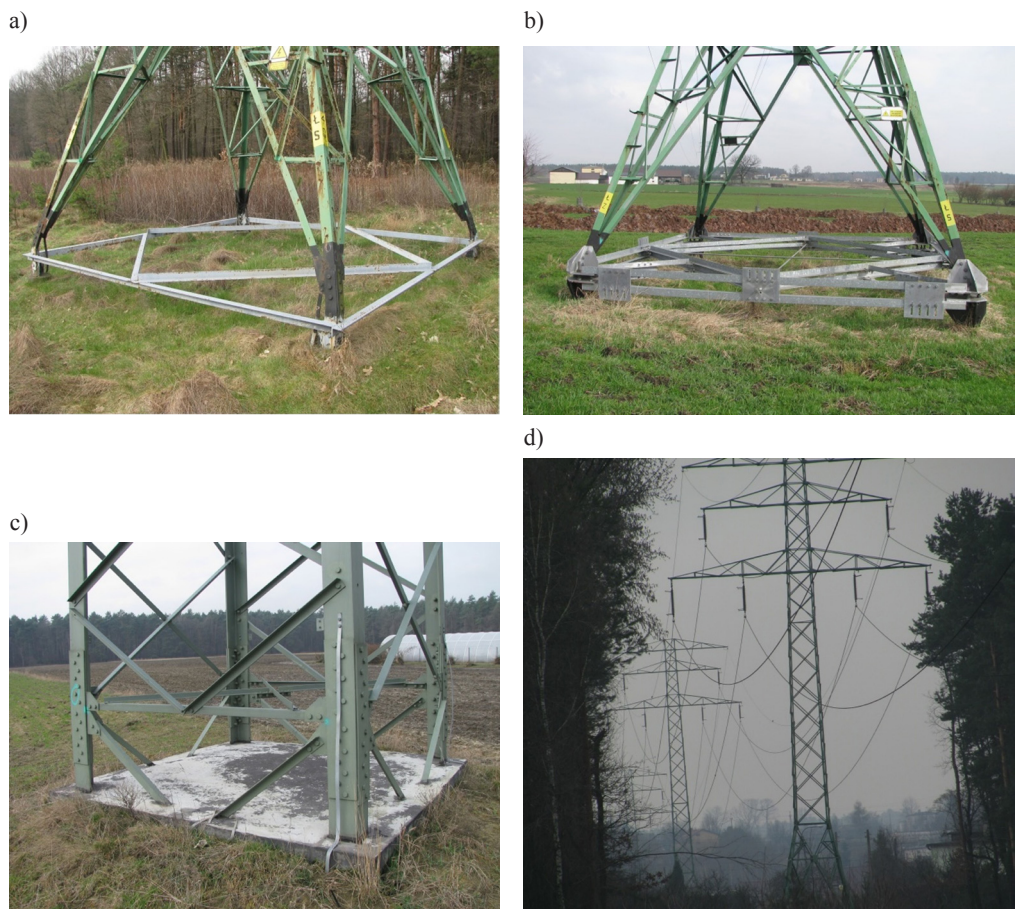
Fig. 8. Examples of repairs of electric power line: a) bracing of the pylon leg, b) bracing of the leg with the possibility of restoring the pylon to the vertical; c) total replacement of the transmission pylon and its foundations; d) regulation of tension stringing of electric conductors
