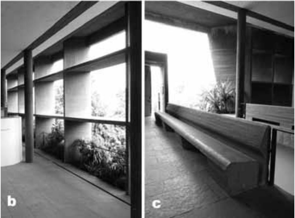
III. 4. Le Corbusier, combining climatic and cultural conditions, introduced the *brises-soleil* on the west façade in the facility of the Mill Owners' Association in Ahmedabad, India (1951–54). On one hand, the concrete grating with diagonally shaped surfaces protects from excessive sun penetration and passers-by, on the other, it distributes air and models the facade with light, photo: autor, 2015
