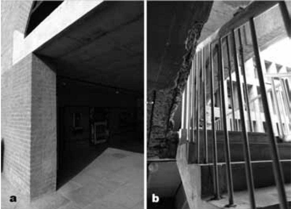
Ill. 2. The performance imperfections in the main building of the Indian Institute of Management in Ahmedabad in India (Louis Kahn, 1961) have caused numerous cracks in reinforced concrete, including brickwork (photo: autor, 2017)
