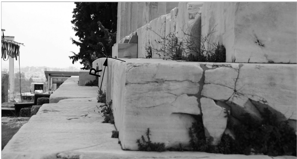
III. 1. Optical correction in part of the Parthenon stylobat, Athen, photo by author, 2010
