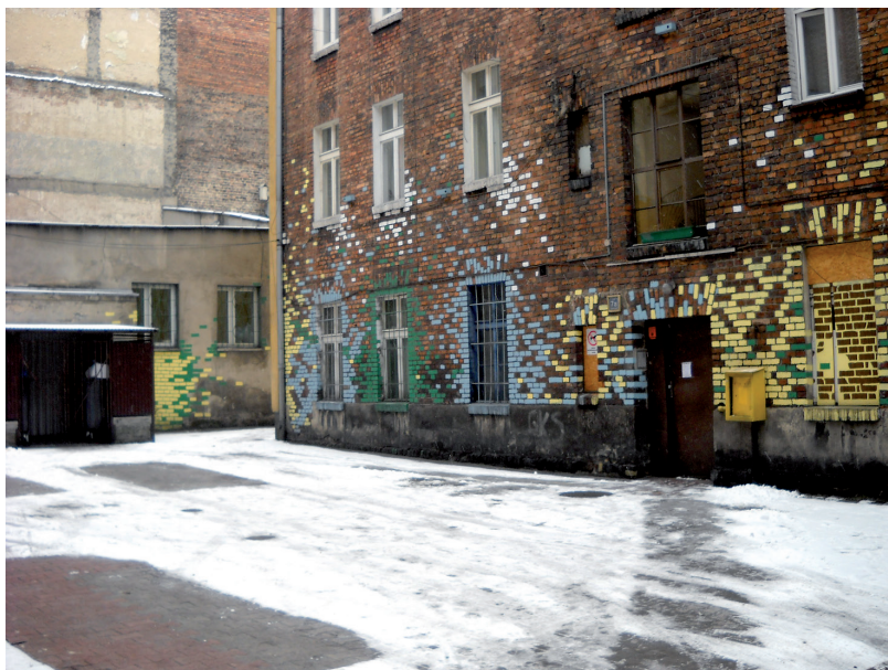
III. 13. One of the three backyards that was upgraded as part of the TAKK project. Some ornaments are left on walls. Traces in the snow show that the backyard is used as a car park. Source: G. Kosmala (2013)
