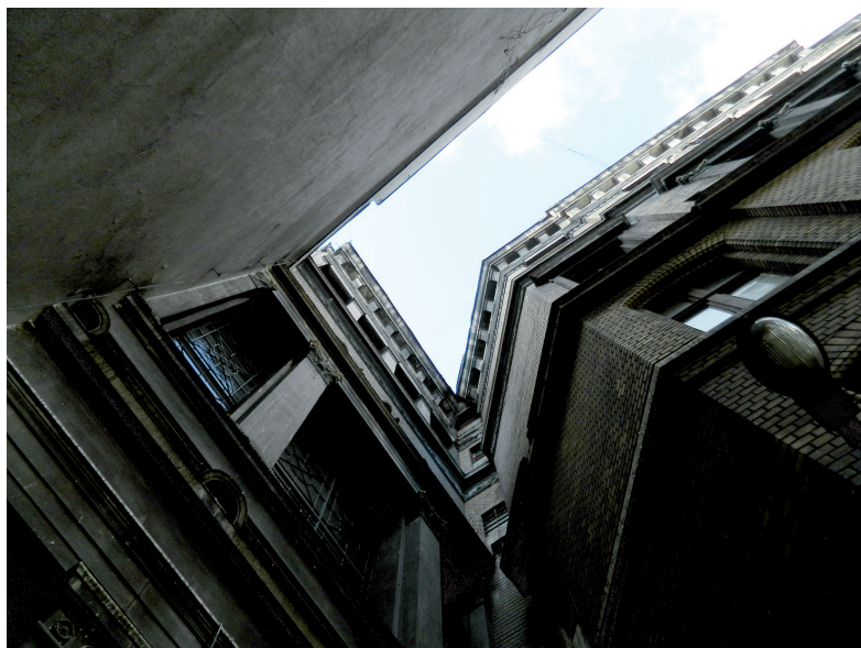
III. 8. A rear, 'hidden' facade of the former Bank of Reich (pl. Wolności 10). Source: D. Chylińska (2013)
