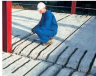
Fig. 1. Steel beam and concrete slabs in Bison project
