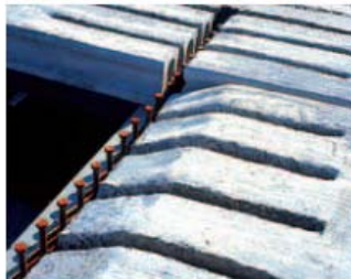
Fig. 1. Steel beam and concrete slabs in Bison project
