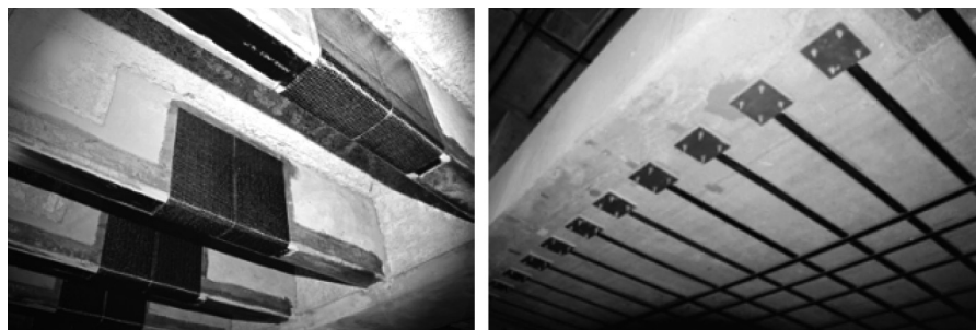
Fig. 1. Examples for strengthening concrete beams and slab with anchoring elements [7]
