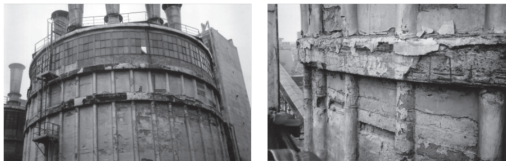
Fig. 4. Corrosion of the prefabricated cylindrical shell (2002)
