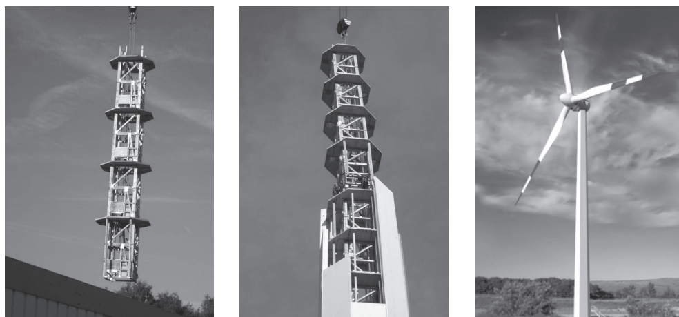
Fig. 3. CLT wind turbine in Hannover (Timber Tower Research Project) [9]
