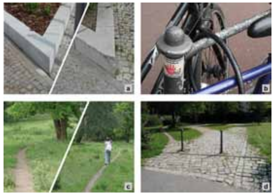
Figure 5: Damage due to design and detailing. a) Damage to acute edging: year 1/year 8. b) Damage to bike stand: year 06. c) Visible signs of use: desire paths: year 7. d) Visible signs of use: year 9
