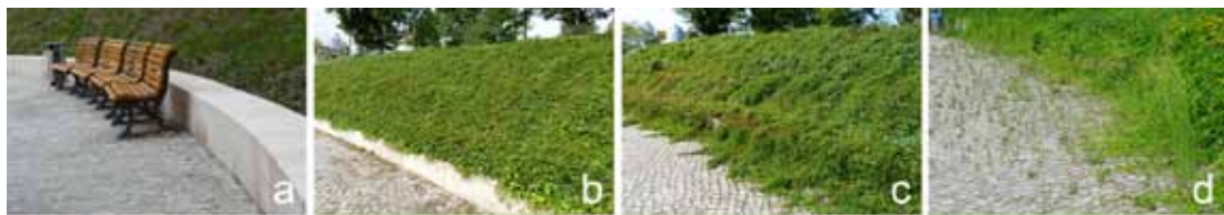
Figure 3: Sequence a-d: The encroachment of planting from embankment onto paving surface over 8 years. a) Year 1. b) Year 2. c) Year 6. d) Encroachment of vegetation promotes further spontaneous growth, Year 8.
