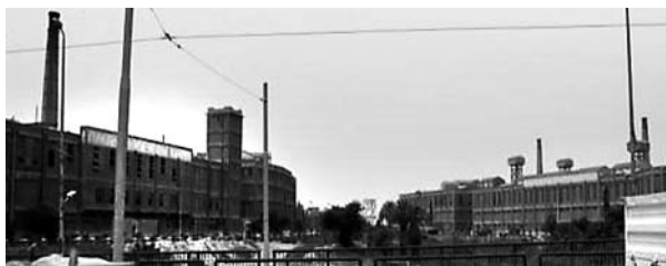
Fig. 8. Panoramic view of the study area on both sides of the canal facing the harbor (Source: authors, 2012)
